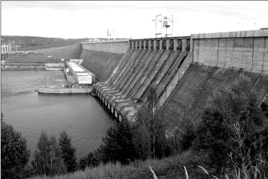
Sarsang Water Reservoir in Agdere
